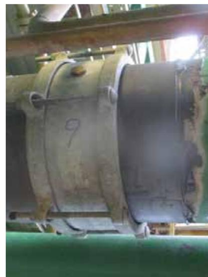
Engate reparado e reinstalado
